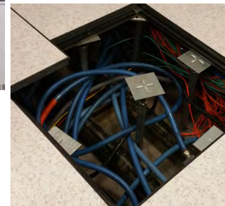
Exposed equipment makes it vulnerable to accidental damage from leaking pipes, fire damage, and spills. A power distribution module is exposed to water and sewage lines above it (photo, above) and a battery backup power unit still shows sign of a recent fire (above, right). Electrical lines are exposed beneath floor boards without any protection from accidental liquid spills (right).
